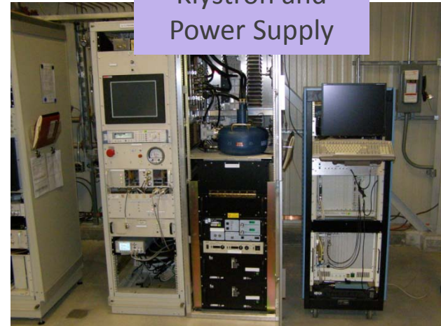
High-power rf system and clean room
