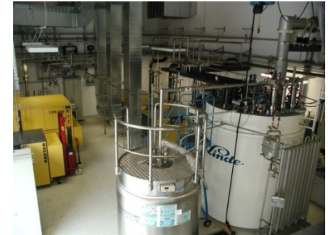
ELBE compressors, coldbox ELBE compressors, coldbox
