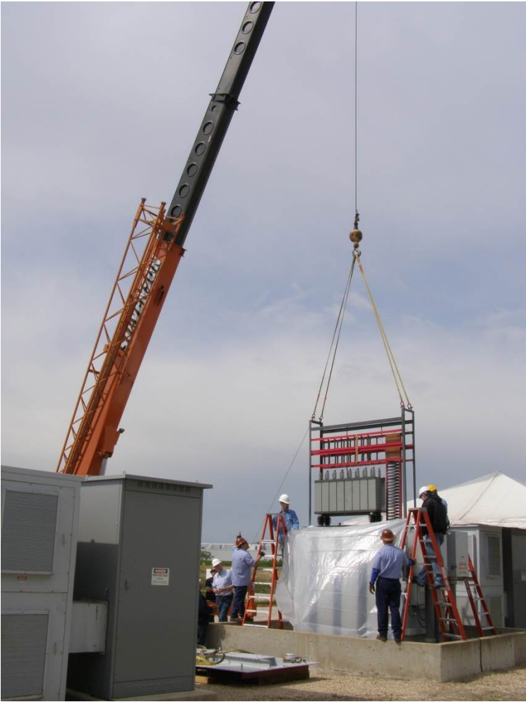
TR Set capacitor bank removal.
