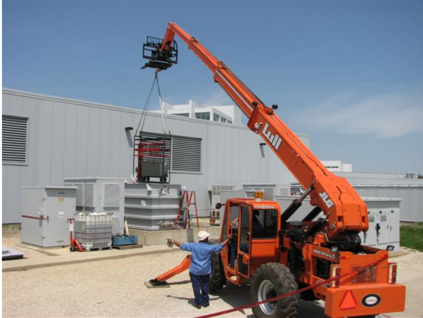
REPLACEMENT OF ORIGINAL T-R SET FILTER BANK CAPACITORS
