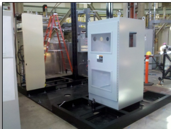
Seismic Base Construction & Cabinet Installation at New Site #2
