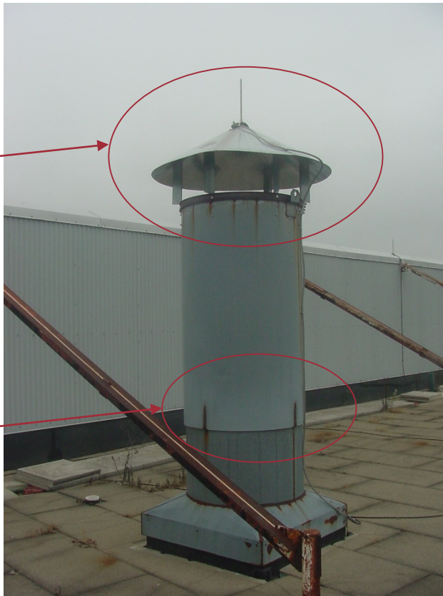
Before sheet metal cap and band were installed
