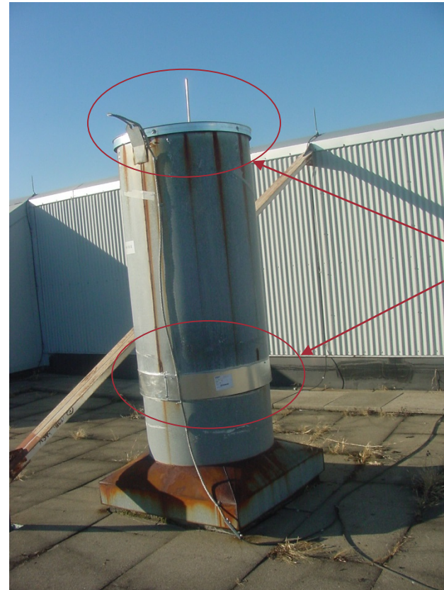
After sheet metal cap and band were installed on Dec 3 2015
