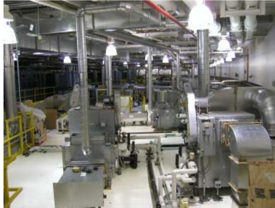
New Ductwork
