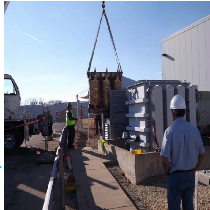
NEW TRANSFORMER INSTALLATION – Feb 1 st , 2016
