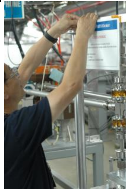
Attaching LOTO signage
