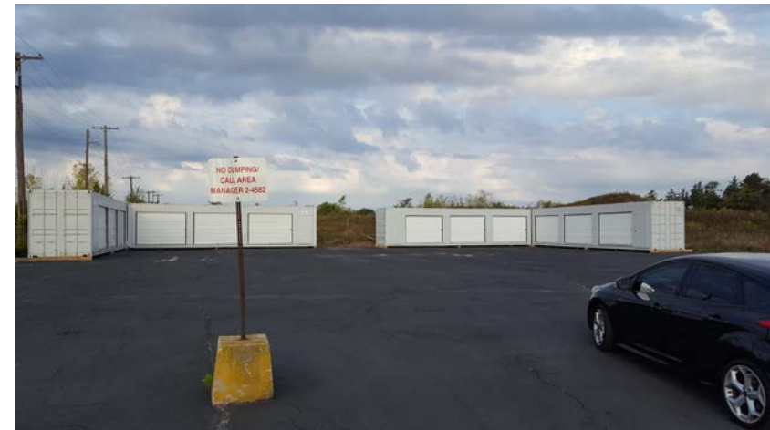
Below: New space in 800-Area for modular containers with roll-up doors
