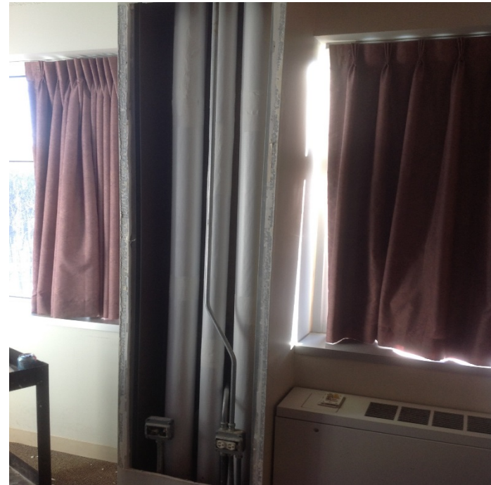
After: New piping fully installed and insulated
