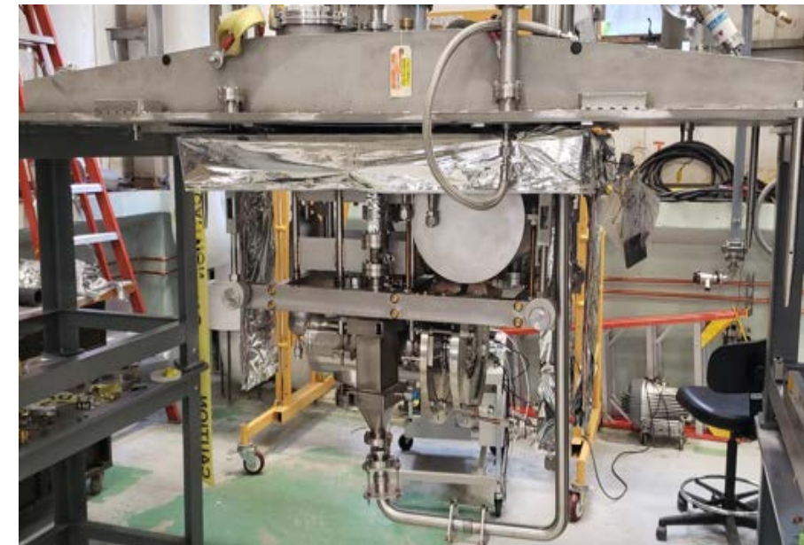
Initial trial fit and check of the bunch lengthening system helium circuit
