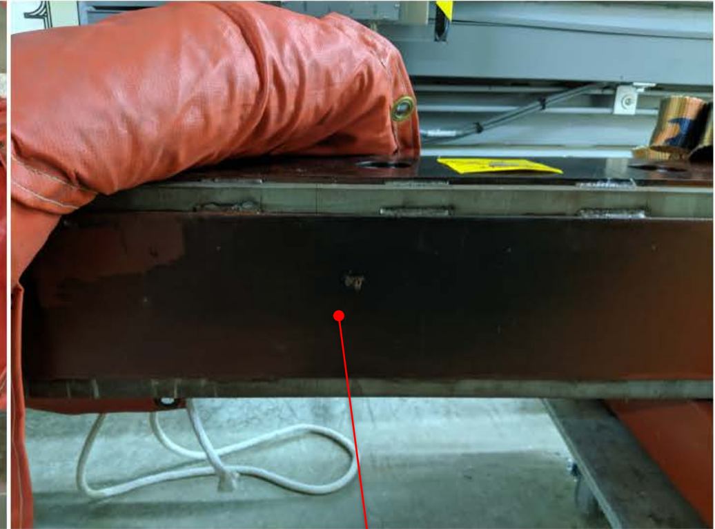
Significant discoloration noticed on side of second failed injection septum
