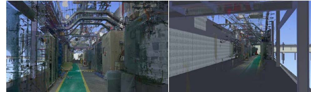
Facility Scans Utilized for As-Built Conditions
