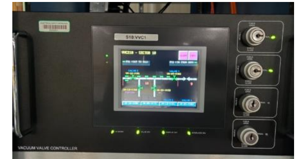
VVC chassis with upgraded CPU processor, power supply, and touchscreen.
