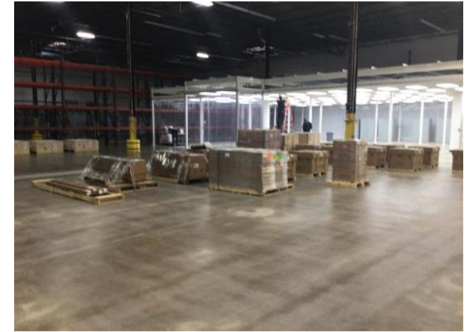
Assembly work beginning at the 981 clean room
