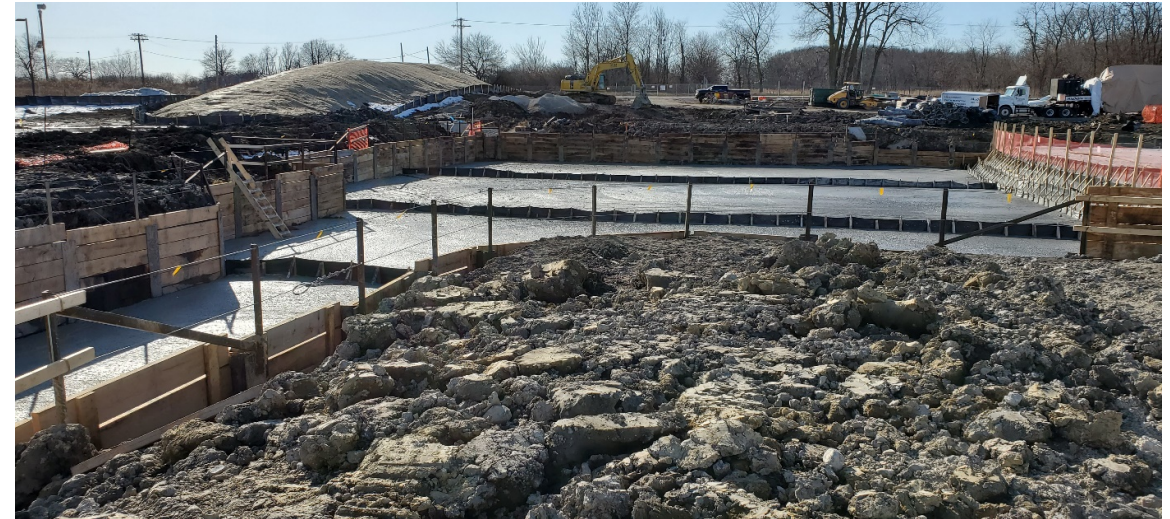
Cellular fill for the ISN corridor and Enclosure area
