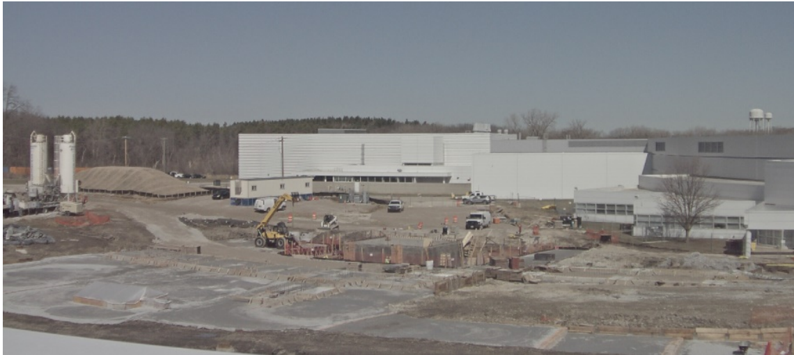
Site Photo from March 19, 2021 showing poured cellular fill
