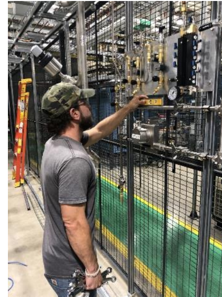
Bunch Lengthening System (BLS) cryo system plumbing in Bldg 420 (left and right)
