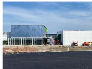
Long Beamline Building progress
