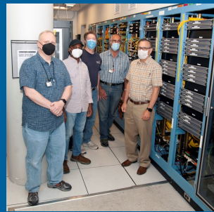
Fiber Shelves in APS Datacenter for the Accelerator, Beamlines, and LOMs
