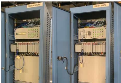
Some of the recently installed temperature monitoring systems
