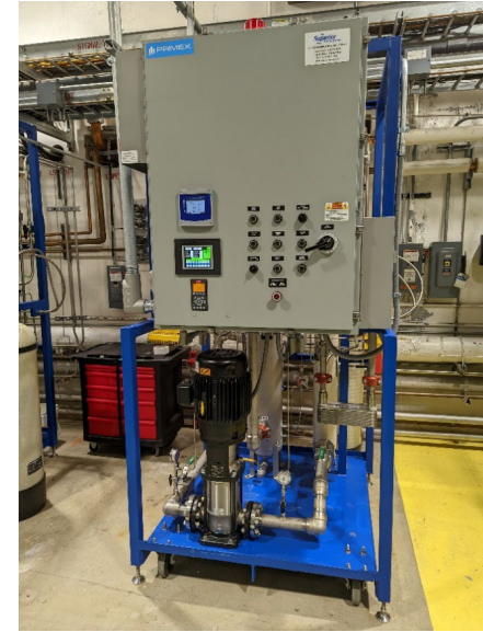
Above right: New L4 water skid
