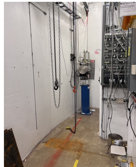
Bend Magnet beamline (5-BM-A) before and after components were removed to prepare for a new wall collimator, utility modifications, and realignment
