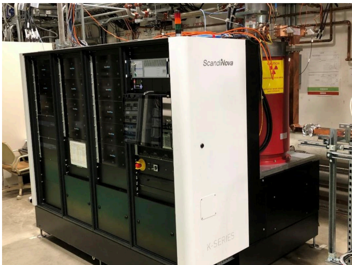
New modulator & Klystron LINAC Addresses obsolescence issues in the APS linac to support APS-U operation
